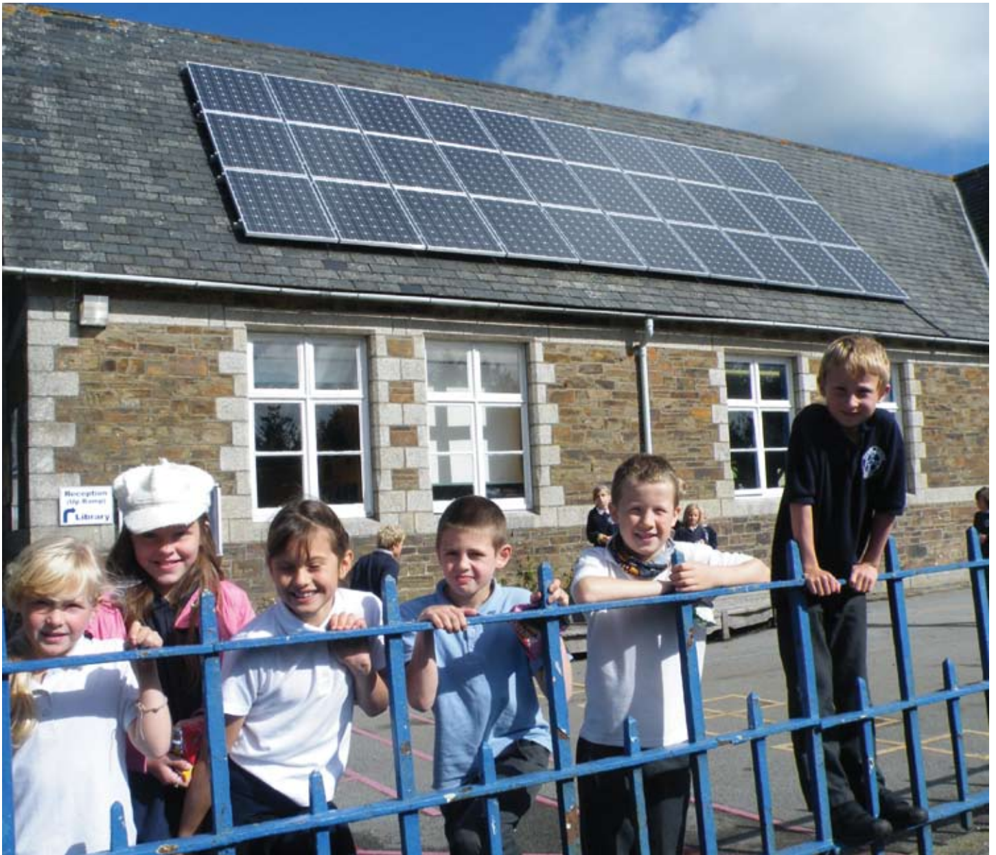
6kWp Solar PV on Upton Cross Primary School
